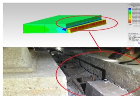
**Figure 12** Instability Characteristics of Track Slab Joint
